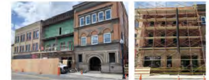
The existing building, pictured in the middle, had been vacant since 2015.
