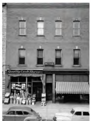
Historic photo of the existing building, circa 1930-1940.
